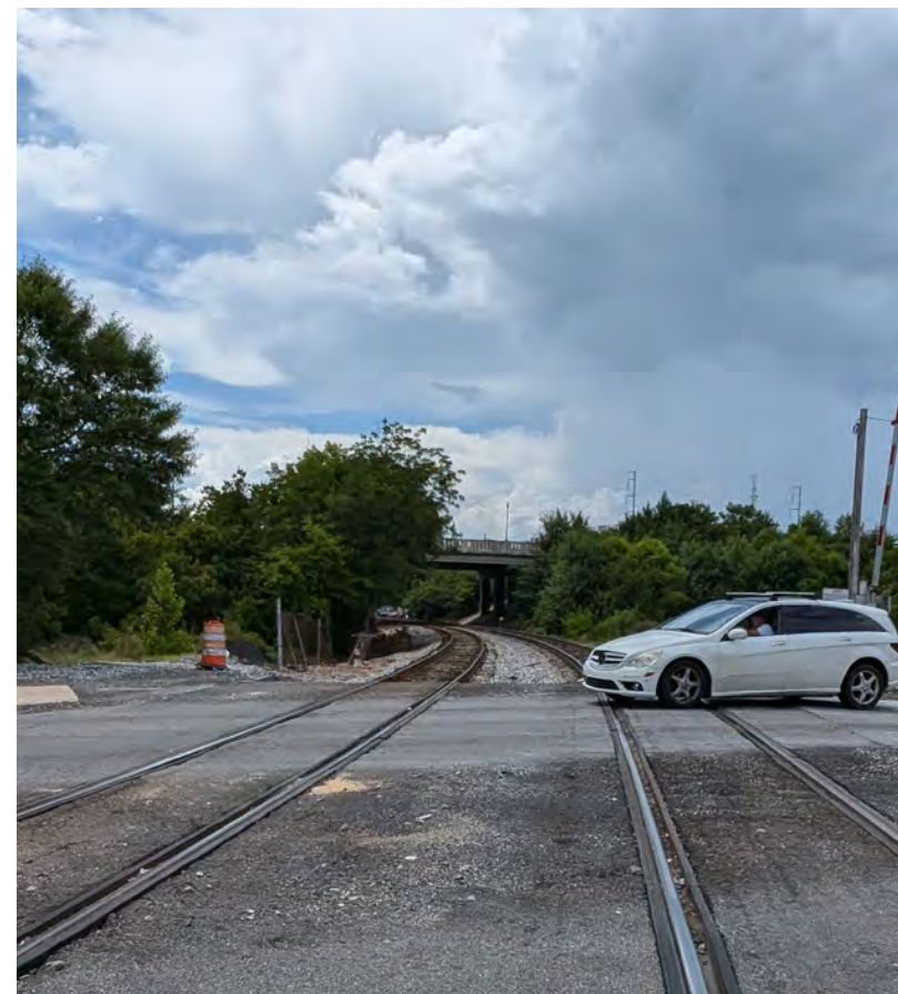
At-grade rail crossing
